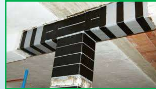
Reinforcement of r.c. elements
