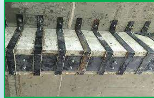
Reinforcement of r.c. elements
