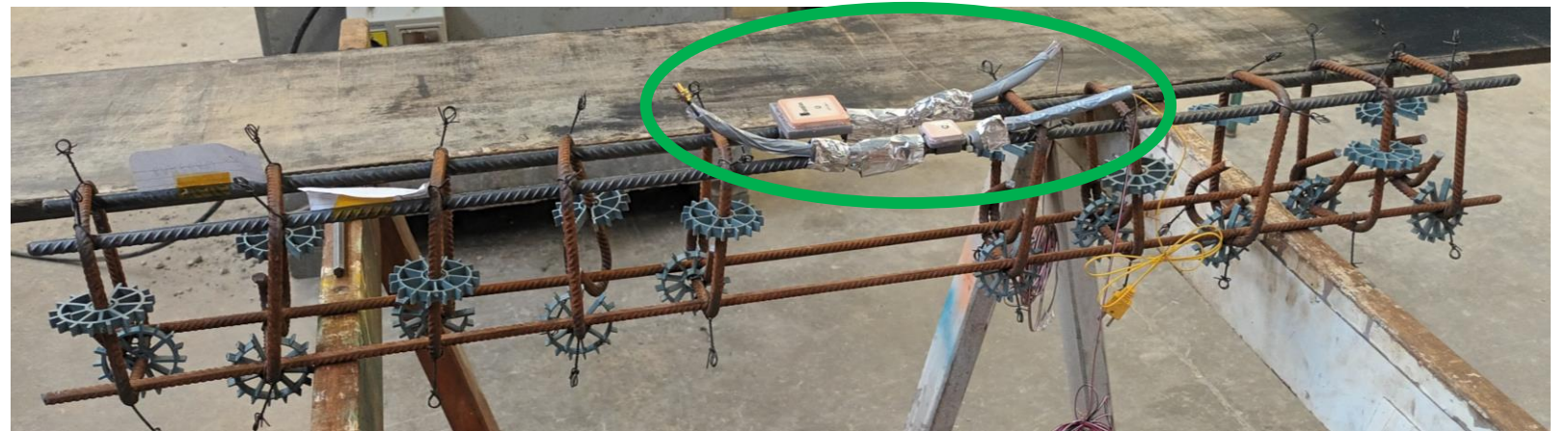
Fig 3 : Metallic reinforcements assembled (upside-down view).
