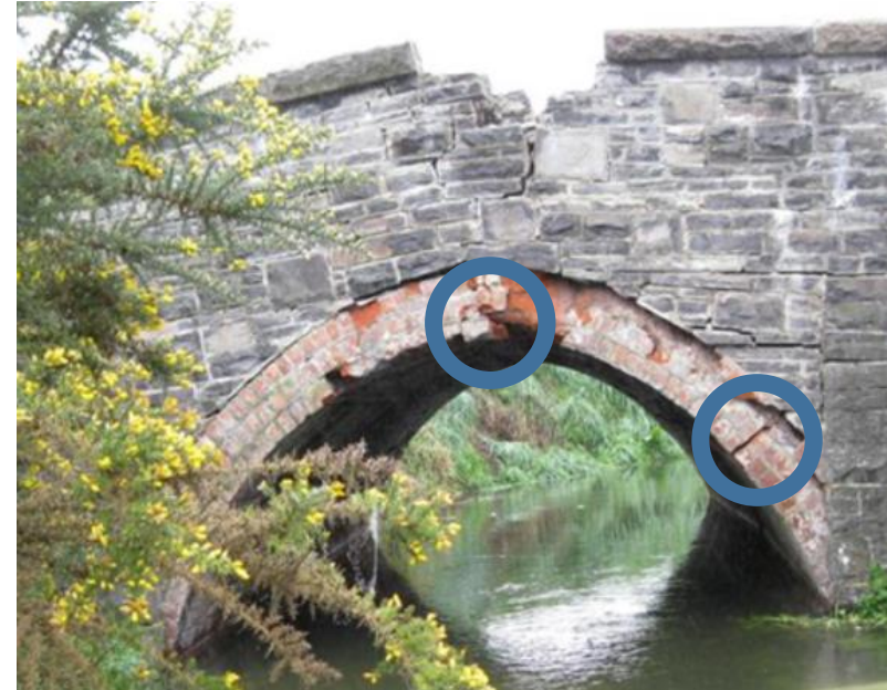
Pedestrian bridge Peru
