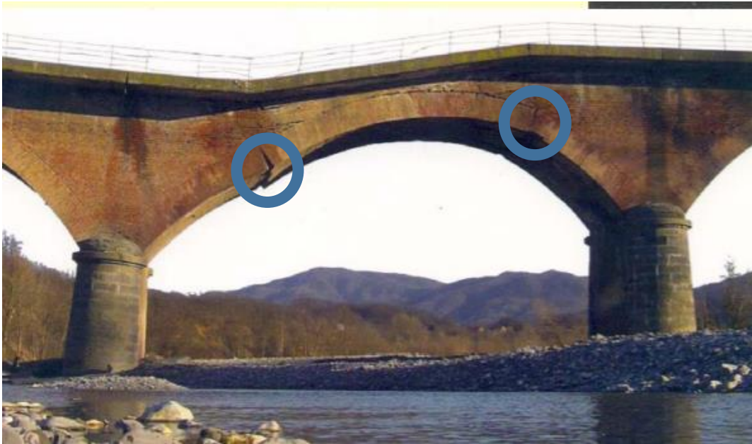
Road bridge Arquata
