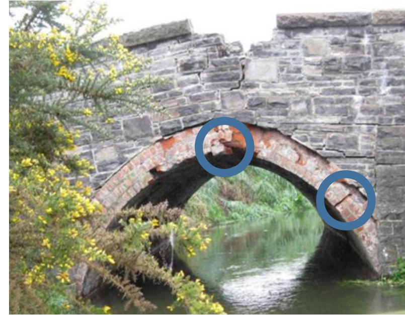
Pedestrian bridge Peru
